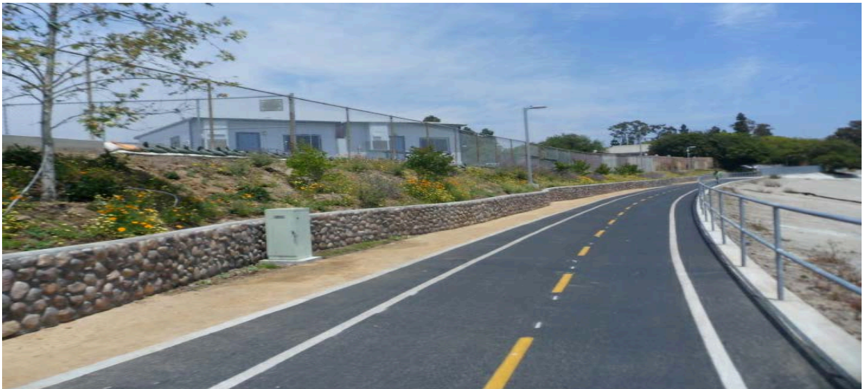
Ballona Creek Bike Path Rain Garden Source: www.culvercitytimes.com
