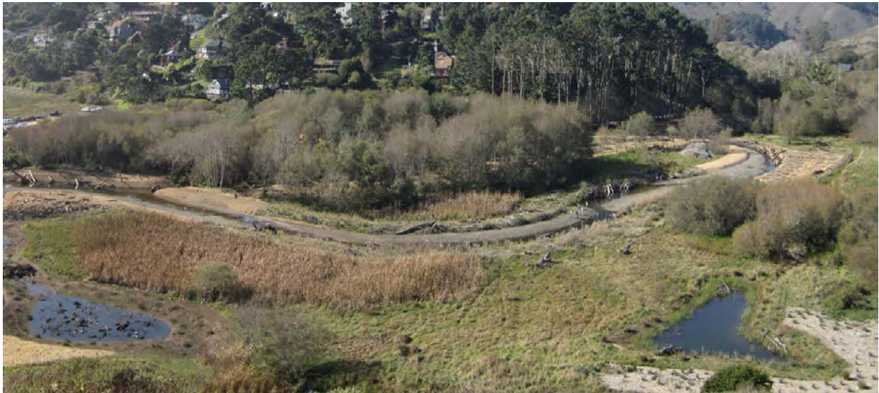
Redwood Creek Post Phase 3 Construction, November 2011 Source: Golden Gate National Parks Conservancy
