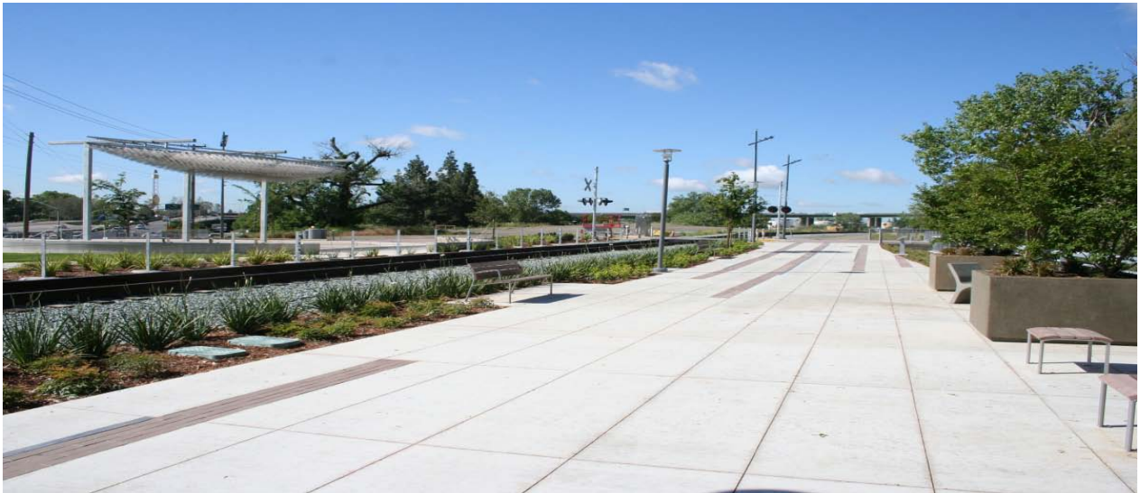
Docks Promenade Parkway—Phase I Source: City of Sacramento
